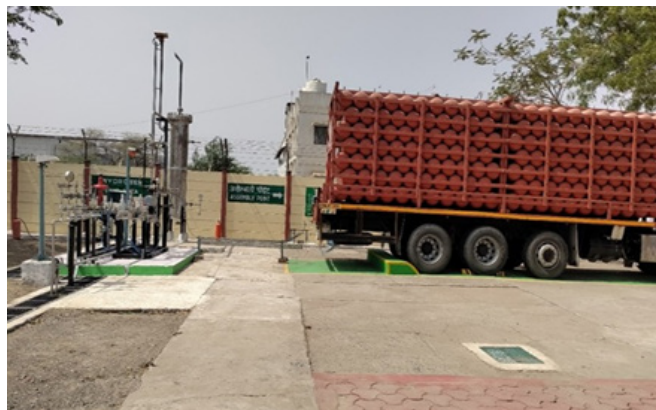
Hydrogen storage cascades with hydrogen pressure regulation skid at City Gate Station of Indore GA of Aavantika Gas
